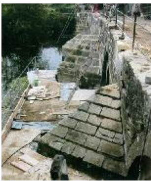
Work underway on the cutwaters during 2003
