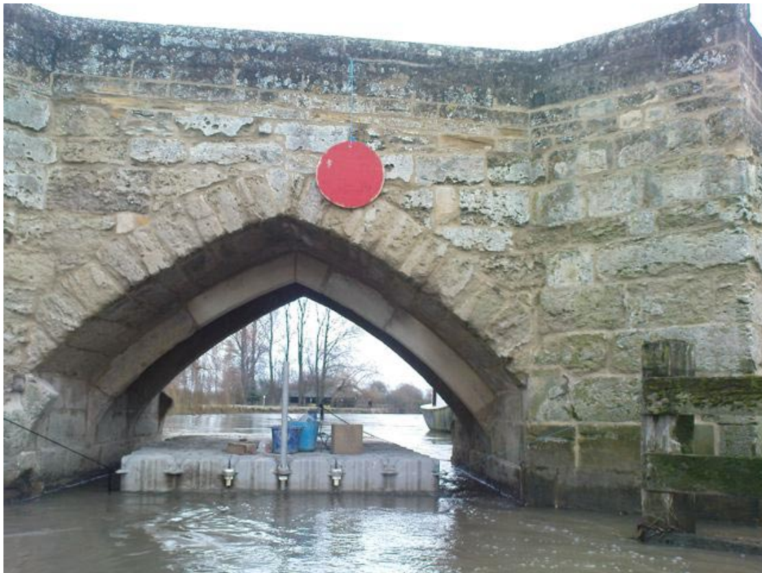
Finished work at Newbridge in Oxfordshire, showing refixed vaulting ribs and completed repointing.
