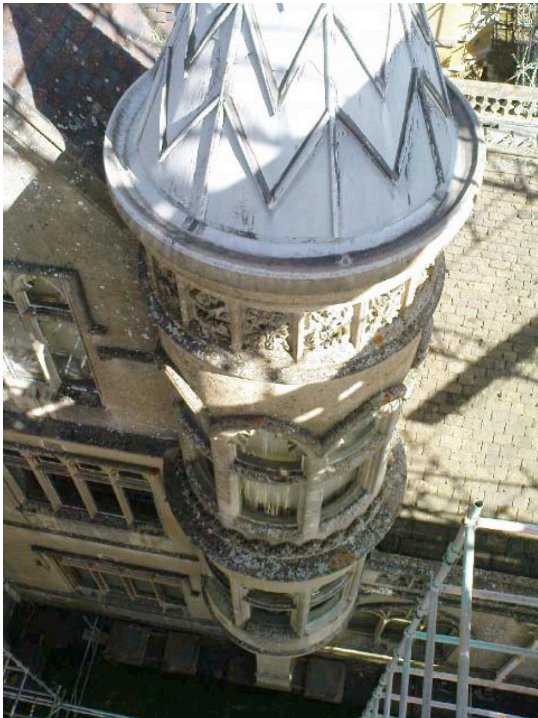
Part of the next phase of works
