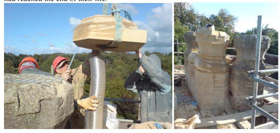
(Above, newly worked Ham and Doulting chimney elements craned into position and nearly finished).
